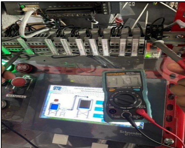
Figure 6. Relay Voltage testing
